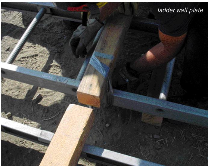
ladder shore strut placement
