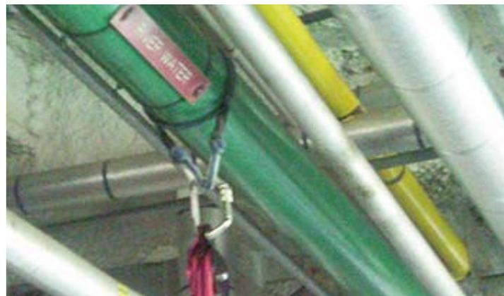
Pipe used for rigging. (pipes to the right were those suggested to be wrapped together)
